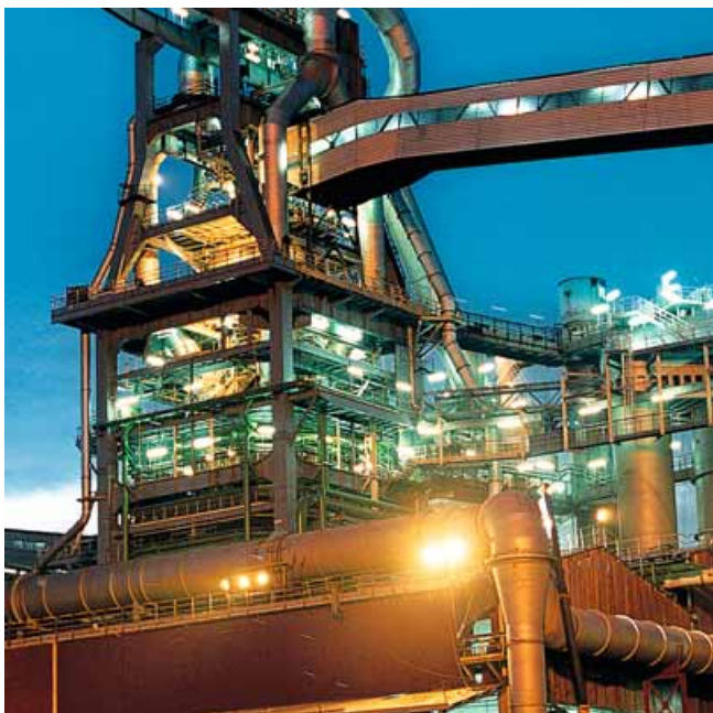
Industrial application: Refinery
